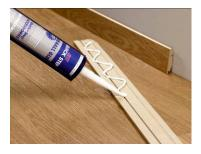
The Quick·Step® ONE4ALL Glue is applied to a clean, dust-free and grease-free sub-surface. Irregularities such as glue residue, etc. should first be removed.
